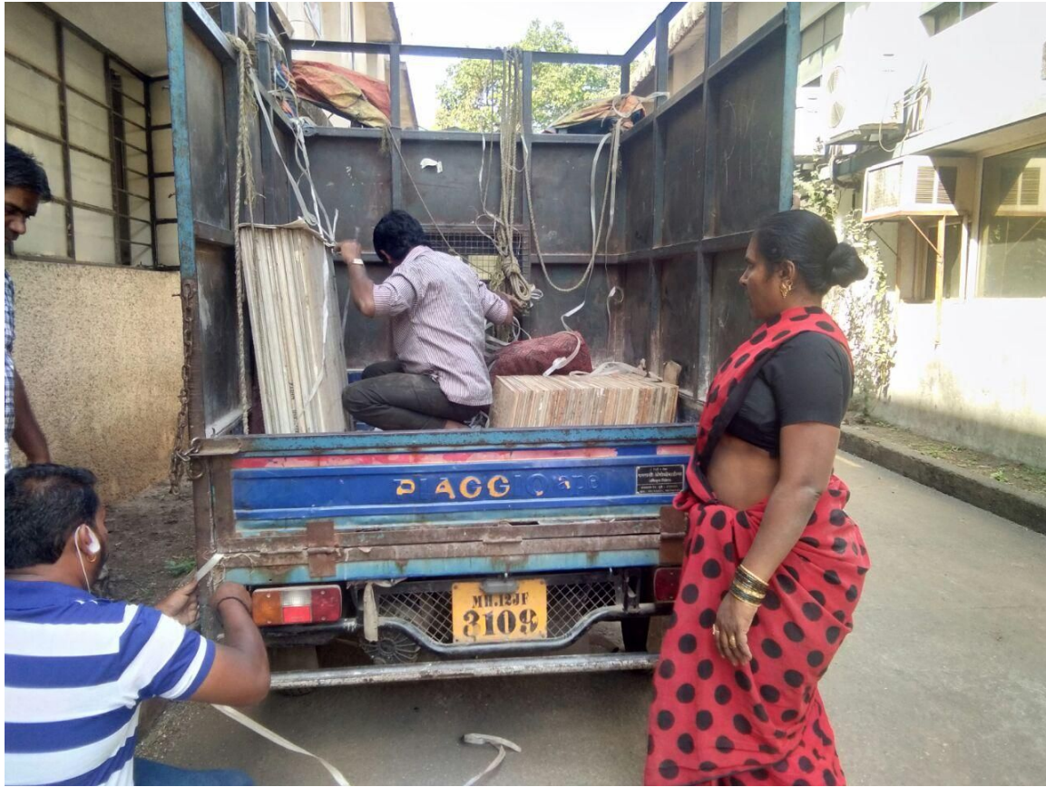
Upgradation of Sarika Shendge's house in Ramtekdi Vasahat, Pune
