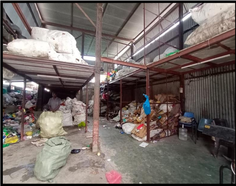
Mezzanine spaces and mesh partitions to optimize space.
